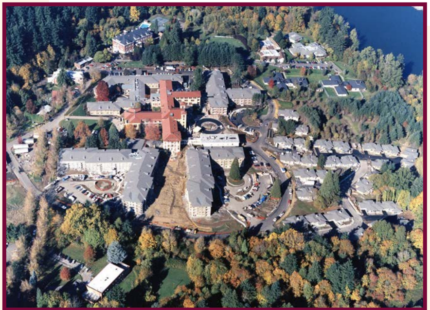
Construction nears completion at Mary's Woods in Lake Oswego (2000). Notice the original SNJM Convent building with the red tiled roof.
